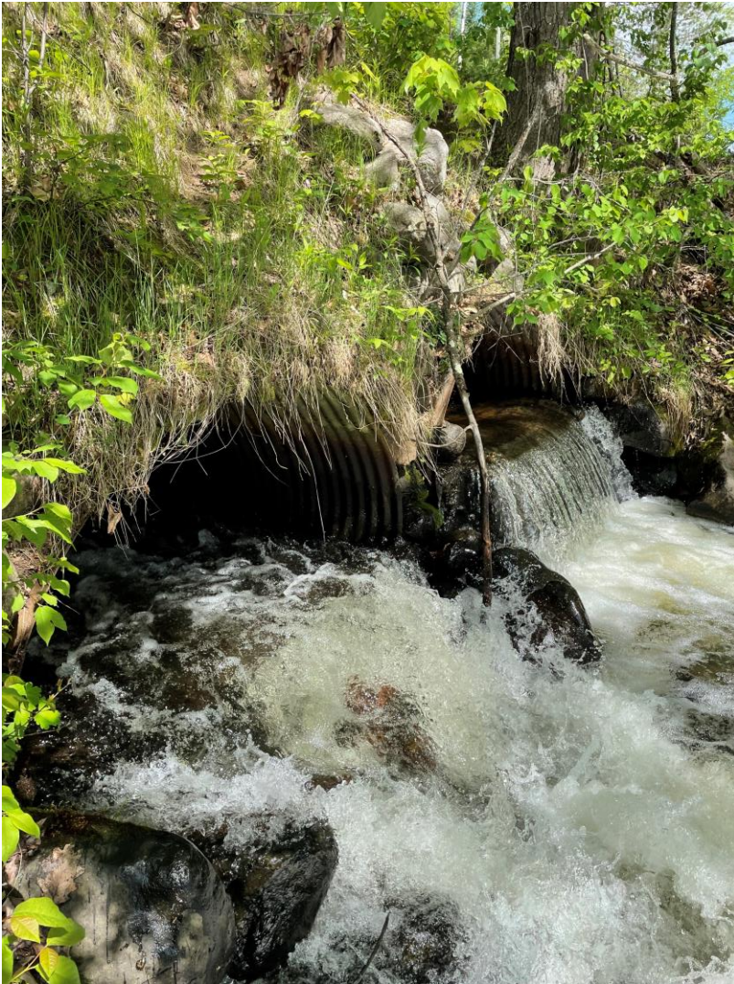
P5: Outlet pipes looking U/S
