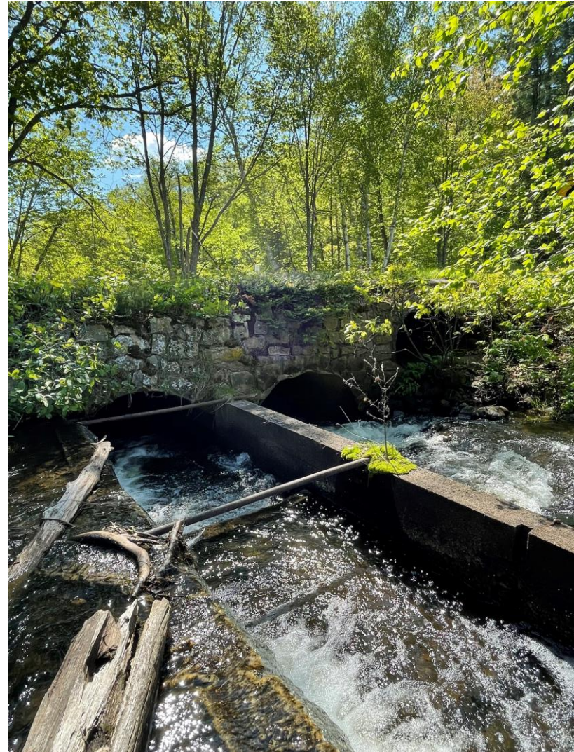
P4: Lower spillway looking D/S
