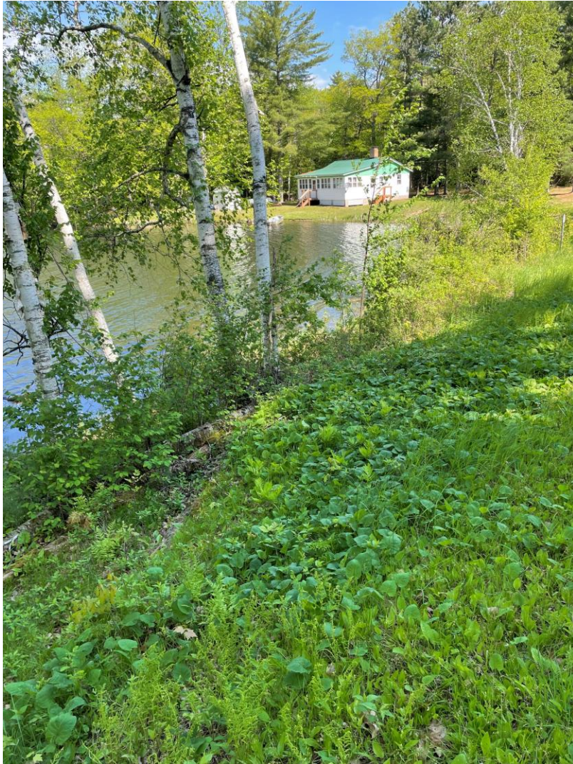
P1: U/S right embankment with woody vegetation
