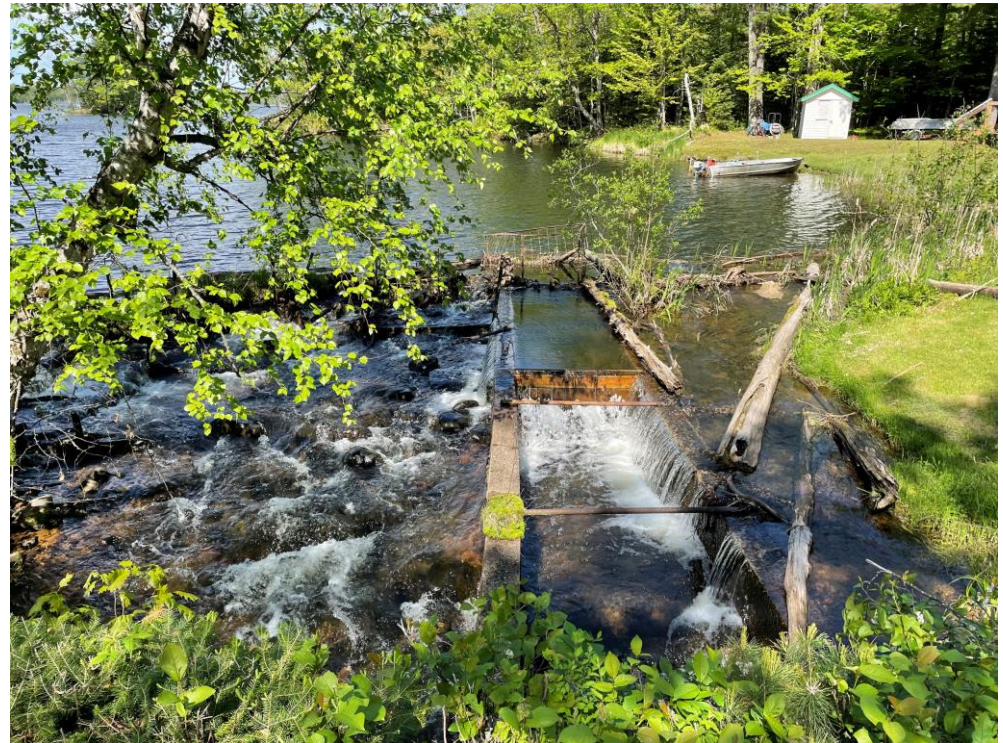
P2: Upper spillway and fishway
